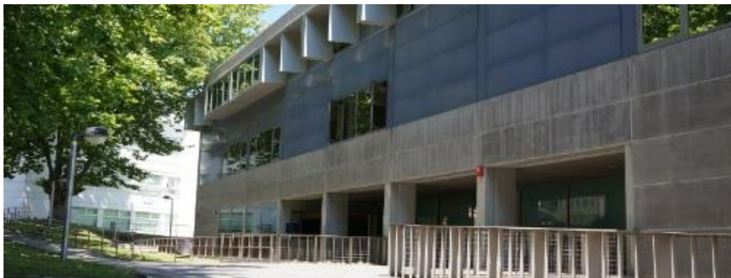
Fig. 4 Exterior appearance of the UDC building used for the example
