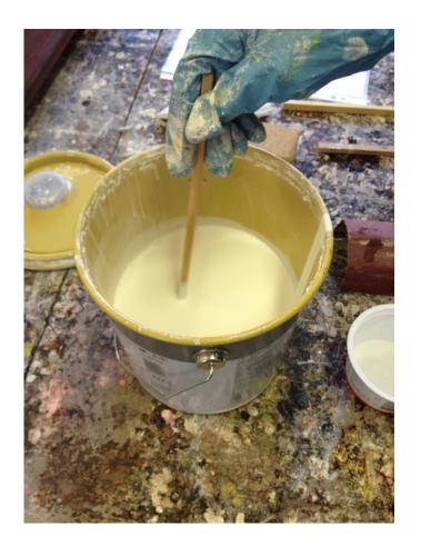
Mix the varnish with the mixing stick all the way from the bottom to the top well.
