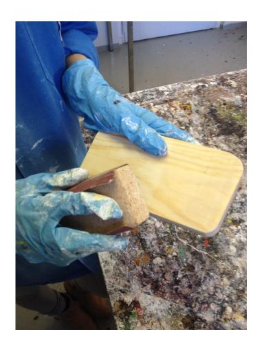
Sand the wood smooth to remove any scratches, lumps or creases with rough sand paper and finish it with the smooth sand paper.
