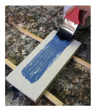
4. Keep the brush in a 45 degree position. Paint parallel to wood fibres.
